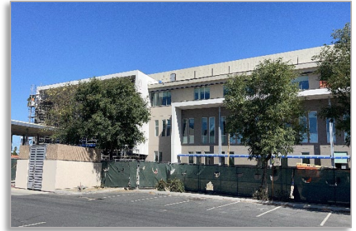
Main Building Exterior
