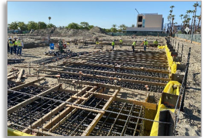
Rebar for Structural Footings
