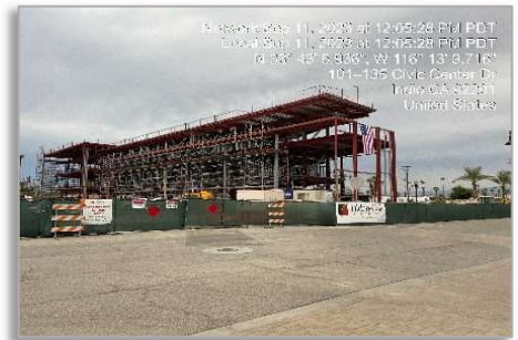
Main Building Steel Erection
