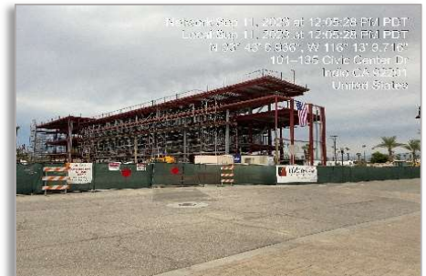
Main Building Steel Erection
