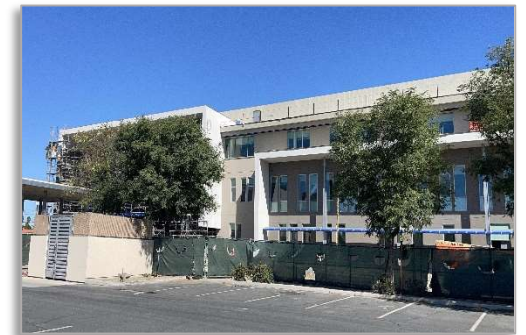
Indio Expansion - Main Building Exterior
