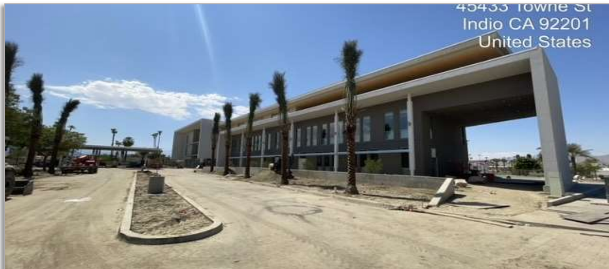
Indio Campus Expansion – Exterior
