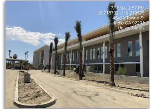
Indio Expansion - Exterior
