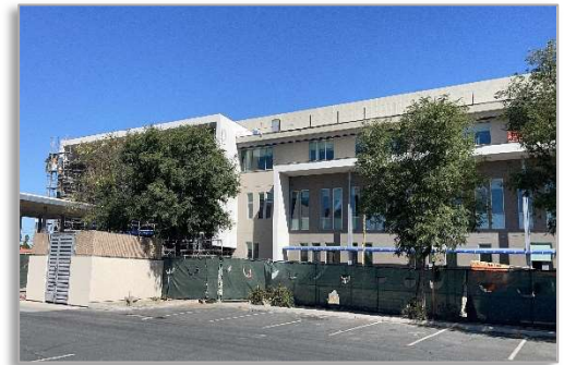
Indio Expansion - Main Building Exterior
