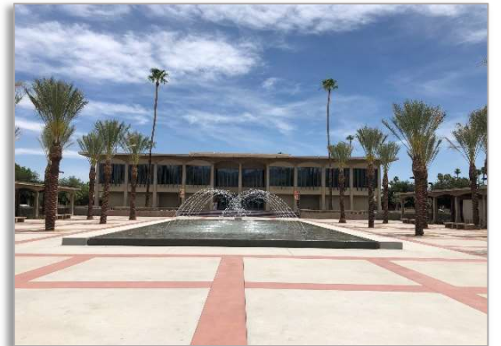
Central Campus Quad towards HILB Building
