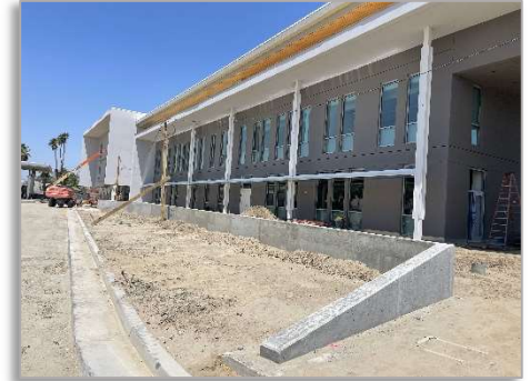
Indio Expansion - Exterior
