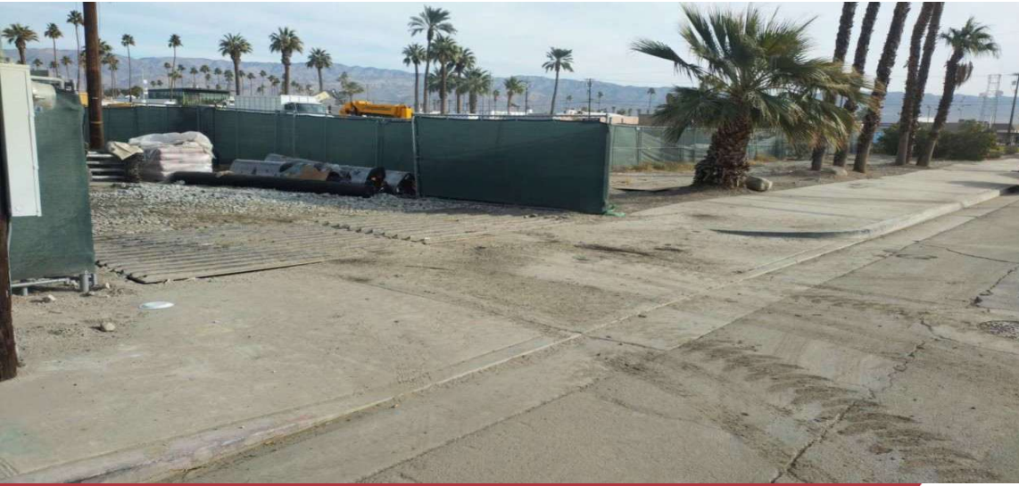
Indio Surface Parking (Construction)
