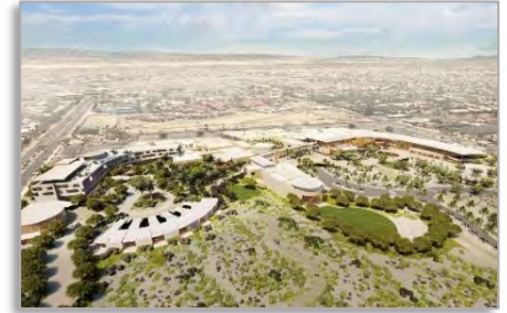
Aerial Site View
