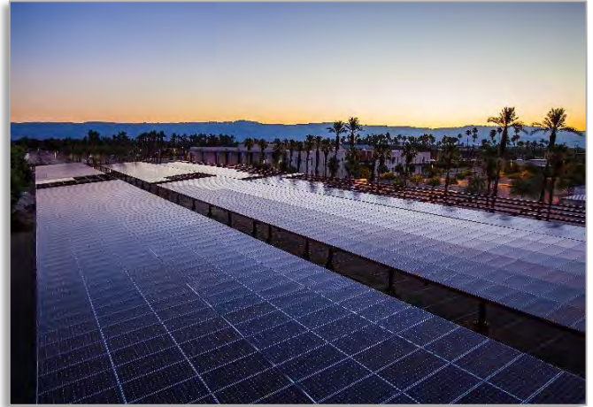
Solar Photovoltaic System
