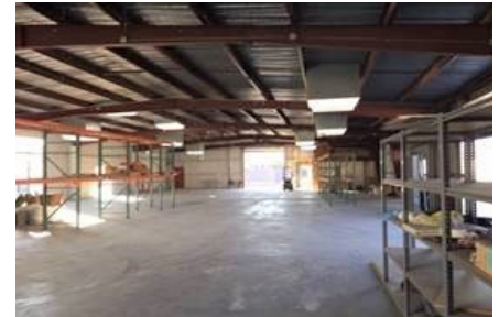
Demolition of Warehouse Interior
