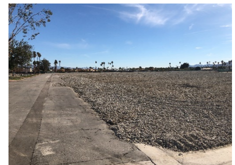
Gravel at Asphalt Transition
