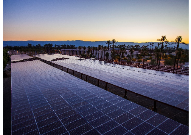
Solar Photovoltaic System
