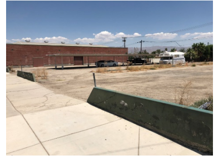
Existing Structures on Site
