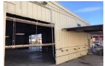
Opening for Custodial Roll-Up Door
